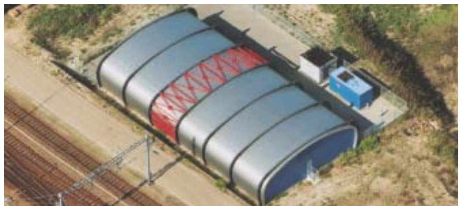
Schakelstation Telfort Amsterdam (NL), 1999. Kalzip® stucco naturel, rond gewalst. Architect: Tebodin 's-Gravenhage
