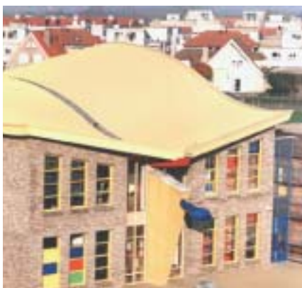
School Culemborg (NL), 1999. Kalzip® RAL 1002. Architect: Anke Colijn Architecten, Utrecht
