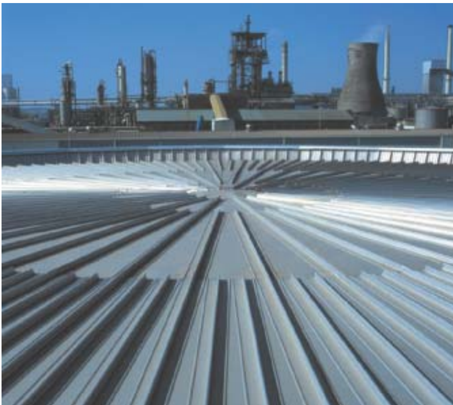
PAC Hoogovens IJmuiden (NL), 1999. Kalzip® stucco conisch. Architect: Saarberg v/d Scheer, Haarlem
