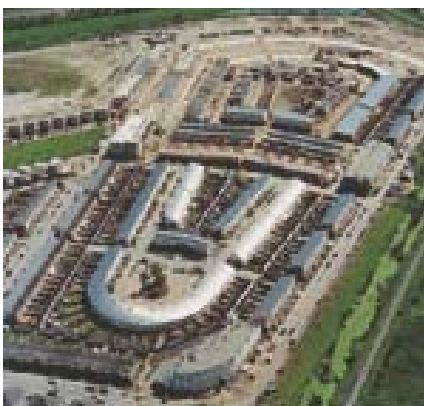
Woningen Alphen ald Rijn (NL), 1995. Kalzip® stucco. Architect: Ronald Knappers, Leiden
